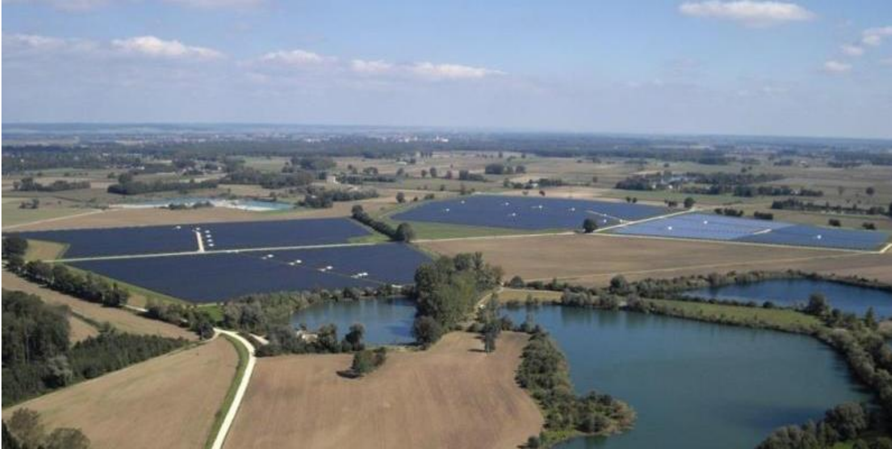
25.7 MW Lauingen Energy Park in Bavarian Swabia, Germany
