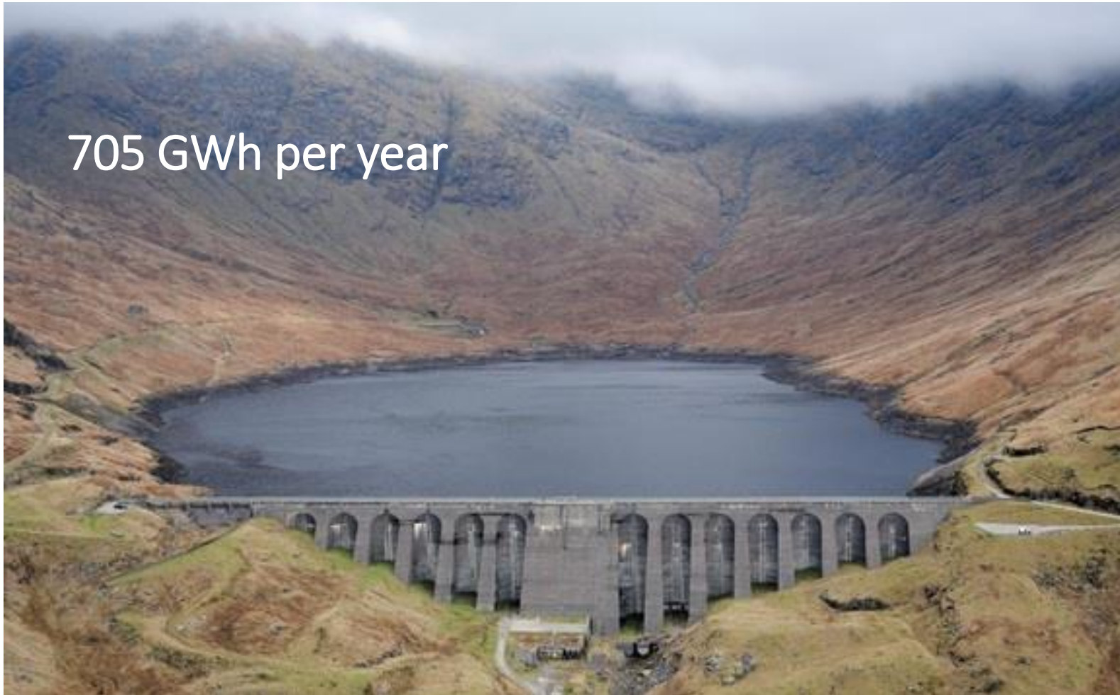
Cruachan Power Station, Argyll and Bute, Scotland
