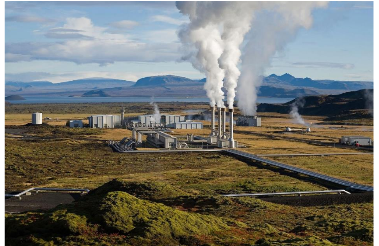
Nesjavellir Geothermal Power Station, Iceland
