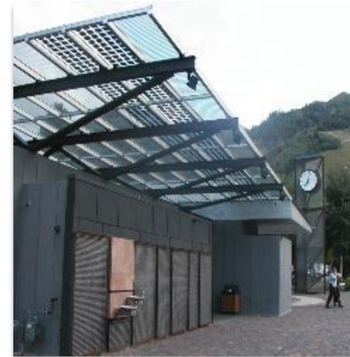
Aspen, Colorado -8 kw - 950 Sq. Ft. - Glass/Glass laminated PV
