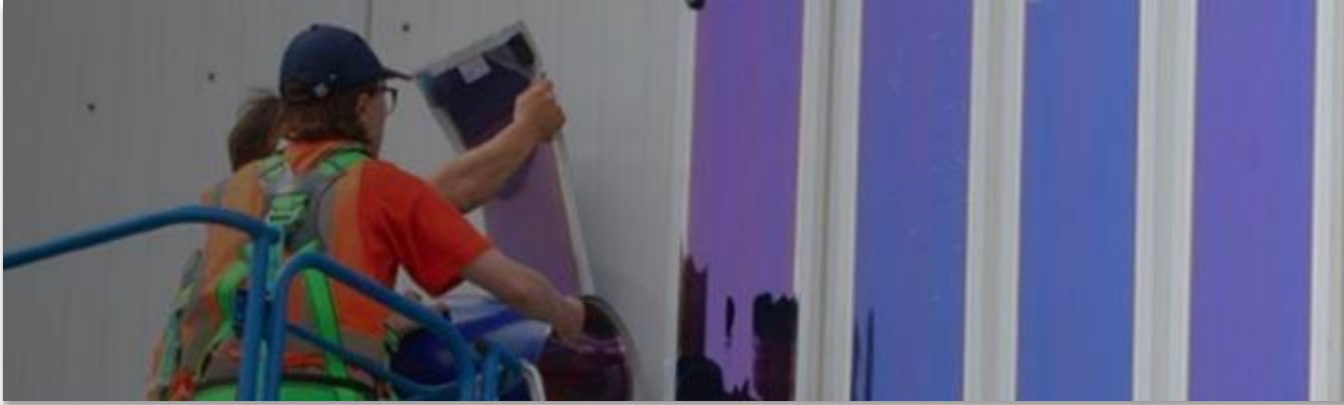
Heliatek being applied to an industrial façade in Germany
