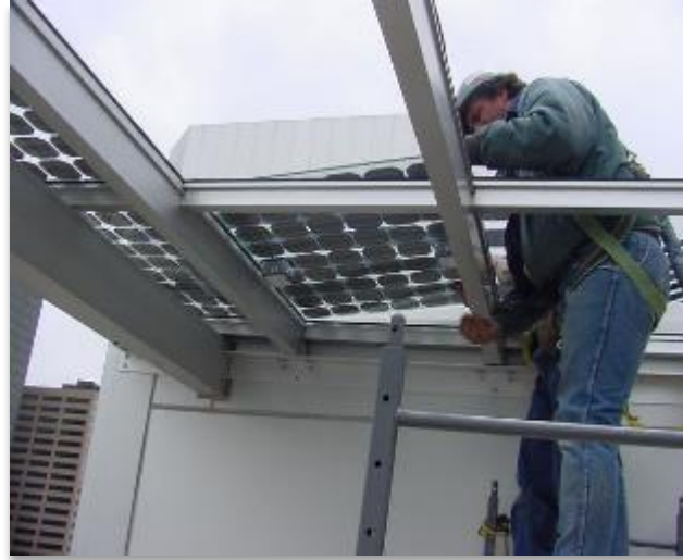
Installation of Laminated PV
