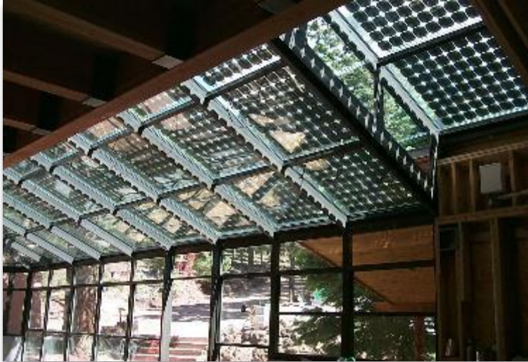
New Mexico - 3 kw -350 sq. ft.- Insulated Glass (Solaria Corp.)
