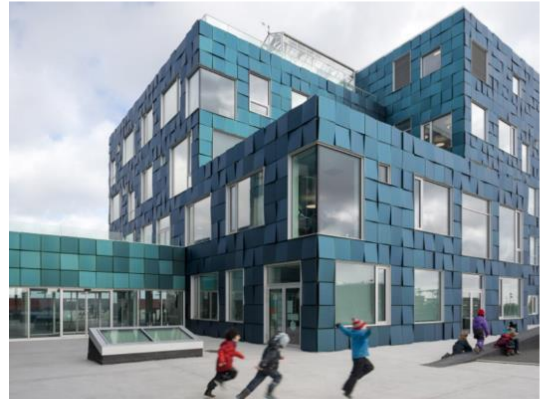
Copenhagen International School, Denmark. Kromatix by SwissINSO. System is 12000 of 0.72m x 0.70m (0.504m 2 ) panels covering 6048 sqm capable of generating 720 kWp (or approximately 119 watts peak per sqm)
