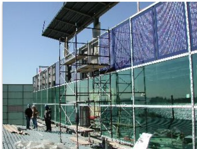
New Mexico - 3 kw -350 sq. ft.- Insulated Glass (Solaria Corp.)
