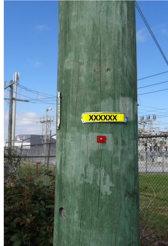
CCA Treated Wood Pole (Green in colour on site)
