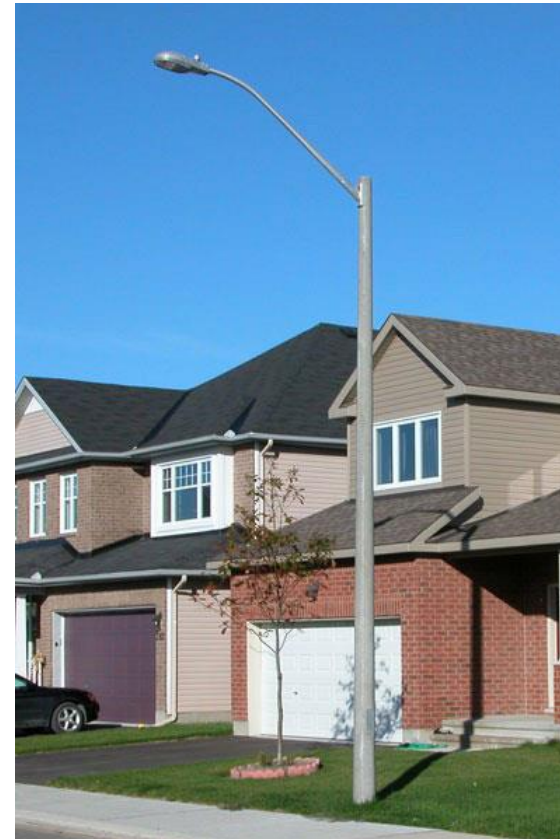
Street light poles
