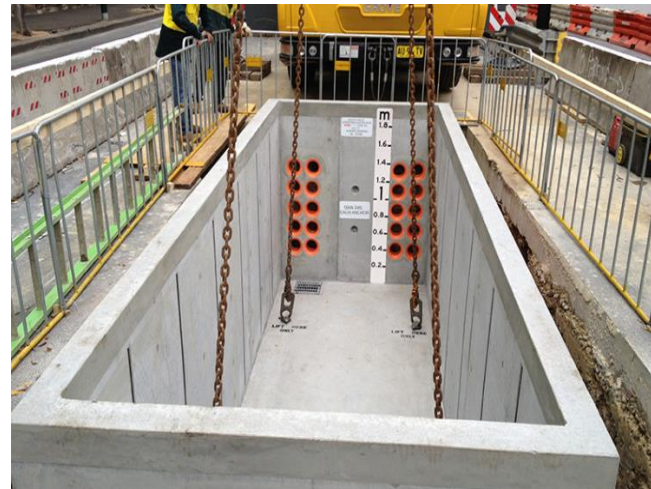
Precast Joint bay lowered to site
