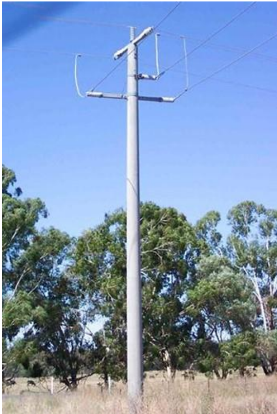
Concrete Pole (Grey in colour & Smooth Finish)
